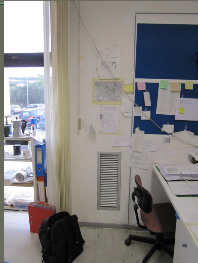
Air outlet in walls
